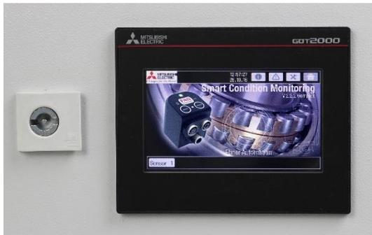
**Image 2:** Mitsubishi Electric's SCM kit provides an integrated approach to monitoring the condition of individual assets and enables a holistic approach to be taken to monitoring the asset health of the whole plant.
